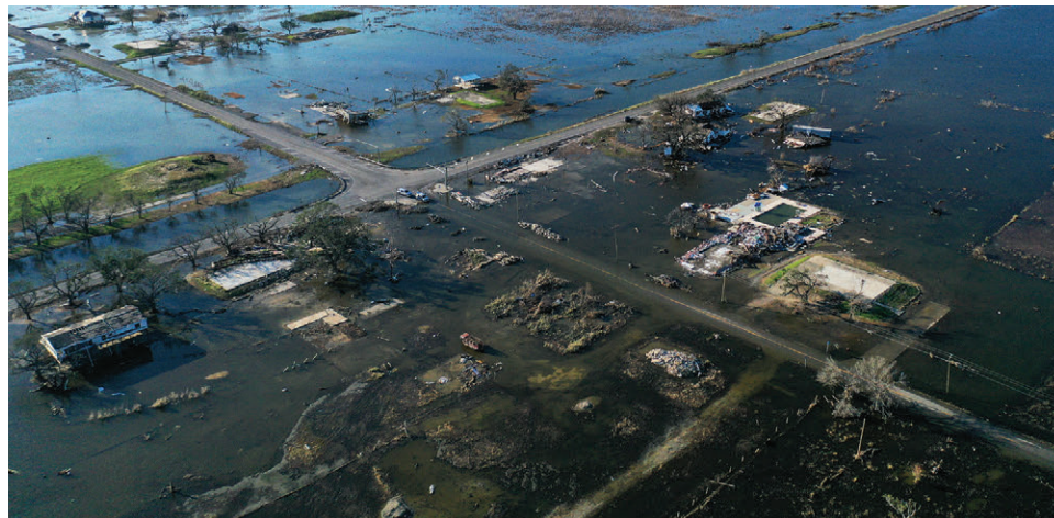
Economic, health and climate change factors help to identify vulnerable communities. Photo: Louisiana coastline after Hurricane Delta.
