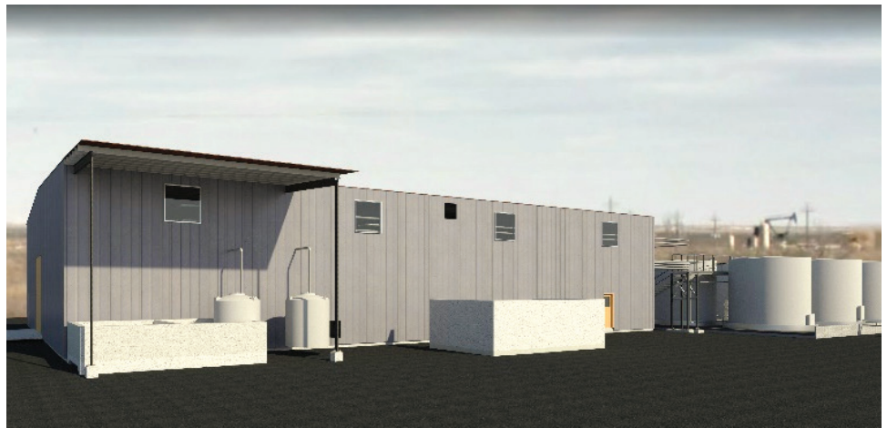
Figure 1: Dynamic Groundwater Recirculation (DGR™) System for Chloride, Hexavalent Chromium, and BTEX. The BIM model for this DGR™ system was developed using Autodesk® BIM 360®, Revit®, Civil3D®, and Navisworks®. The model includes the treatment plant as well as the extraction and injection well networks. The model was incorporated into HoloBuilder™ and used alongside 360-degree photos and a virtual reality headset to facilitate construction using as much remote expertise as possible during the ongoing COVID-19 pandemic.
