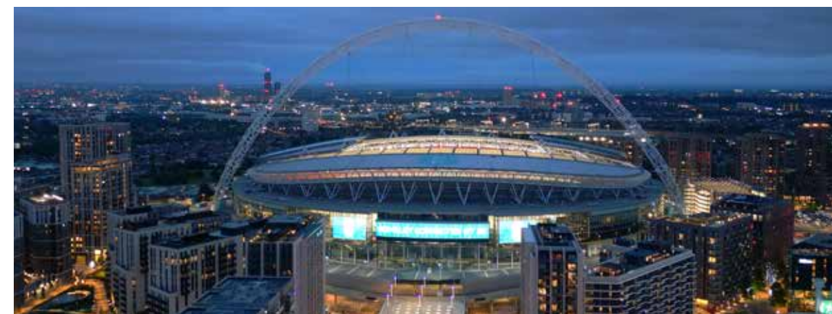
Wembley Stadium London, UK
