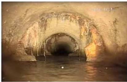
Picture above: Root intrusion into a pipe indicates likely infiltration of clear water and can block sewer flow. NEW Water Televising Program.
